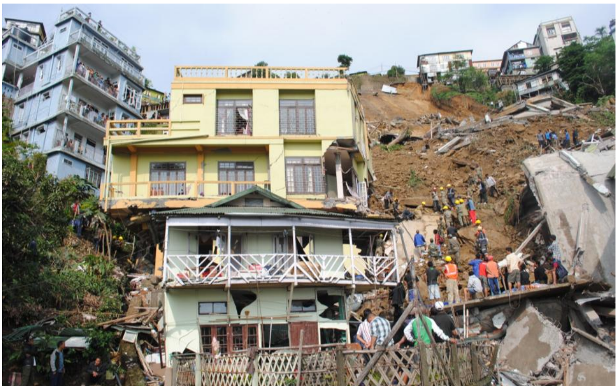
Figure 1. Site and extent of rockslide at Laipuitlang, Aizawl, on 11 May 2013.
